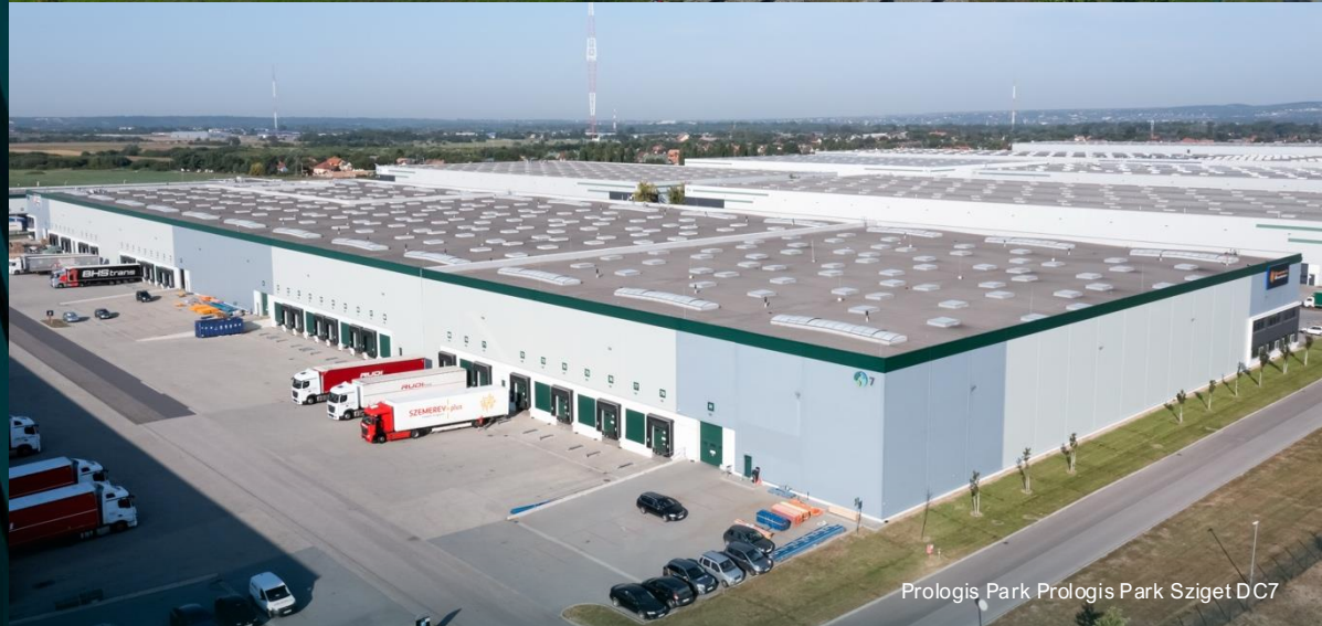
Prologis Park Budapest-Harbor DC9
